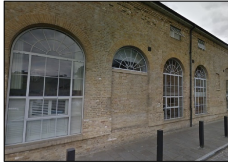
The former Goods Shed has been redeveloped
